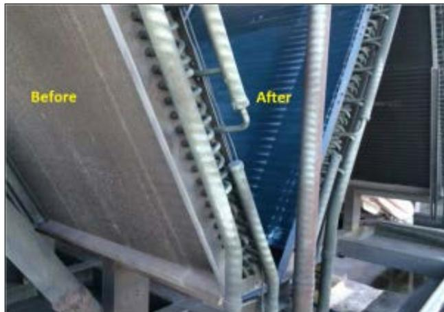
Coil faces showing the completed application of the HVAC Armor product on the inside, vs the non-completed existing exterior coil face that will be coated next outside.
